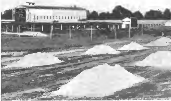
Crushed Surface Rock Ready to Spread on Old Track
